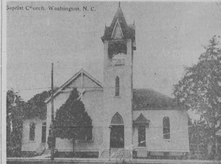
THE FIRST BAPTIST CHURCH of Washington as it appeared in the year of 1900. The church was located on the west side of Market street, between Second and Third streets. Much of the heavy timber of the Free Church was used in the remodeling of the Baptist church in the year of 1896. The church purchased property and moved to its present location on East Main street in 1917.
